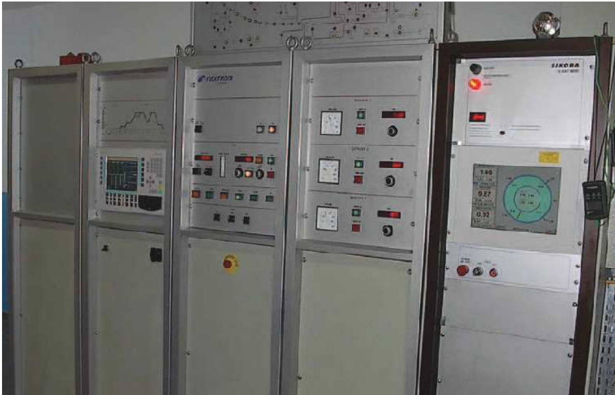
Control Panels show readouts for dimension, temperature, line speed and various other feedbacks
